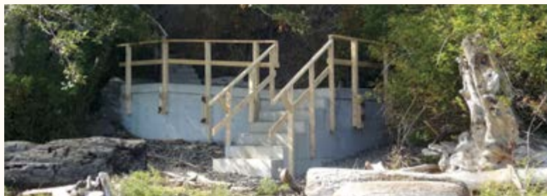
The repaired access to Weir Beach. Allen Jones photo.
