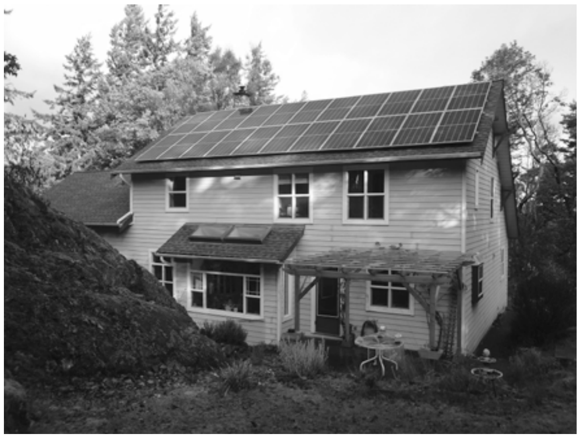
Left: Brendan and Jeff from Shift Energy. Above: solar array to the rear south facing roof.
