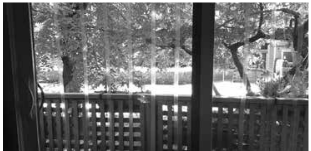
'CollidEscape' tape on glass doors
