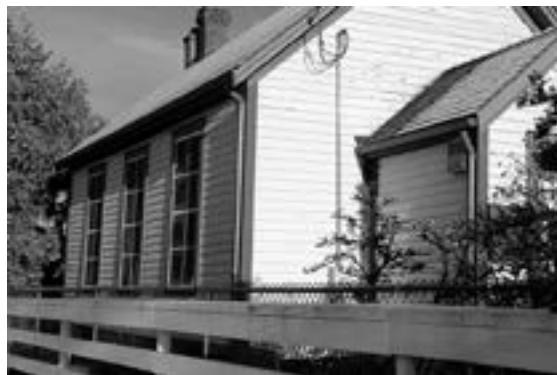
The fine new gutters and down spouts on the School House Museum, generously donated and installed by the Ryan Craycroft family of Network Home Improvements. Brian Domney photo
