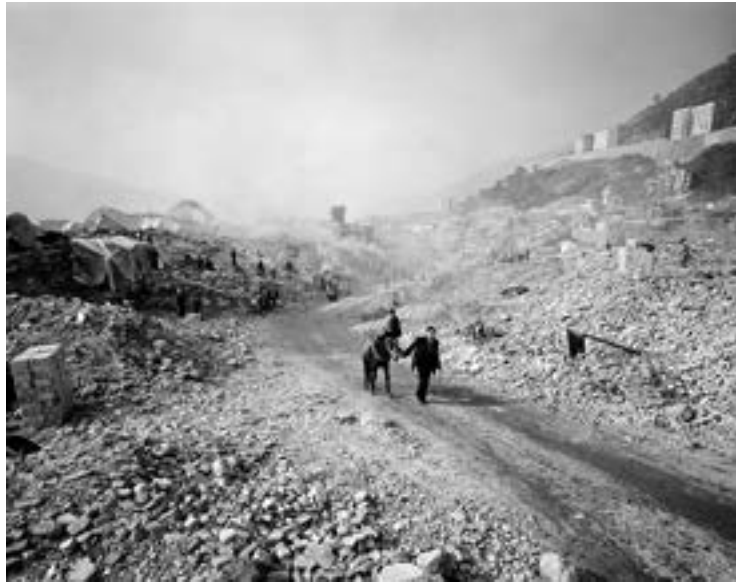
Three Gorges Dam Project, Yangtze River, China.
