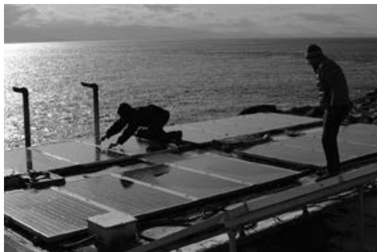
Perron Electrical Installations, working on installing solar panels.
